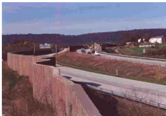
Figure 22. "Zig-zag" barrier photo #8057
