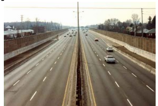
Figure 18. Parallel noise barriers photo #2968
